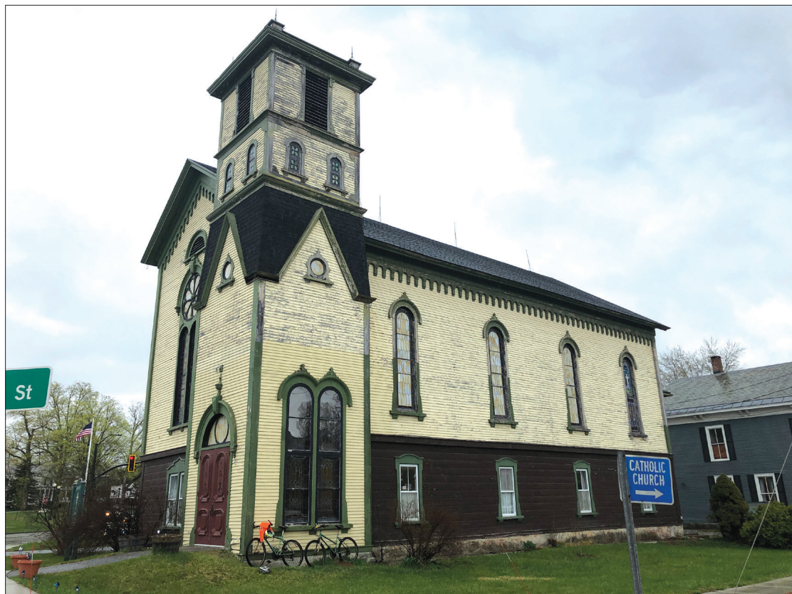
THE BRANDON METHODIST Church has stood at the intersection of Carver and Franklin Streets since the 1870s. The physical maintenance of the building is a daunting task but the congregation has recently replaced the roof and is working to obtain further grants.
